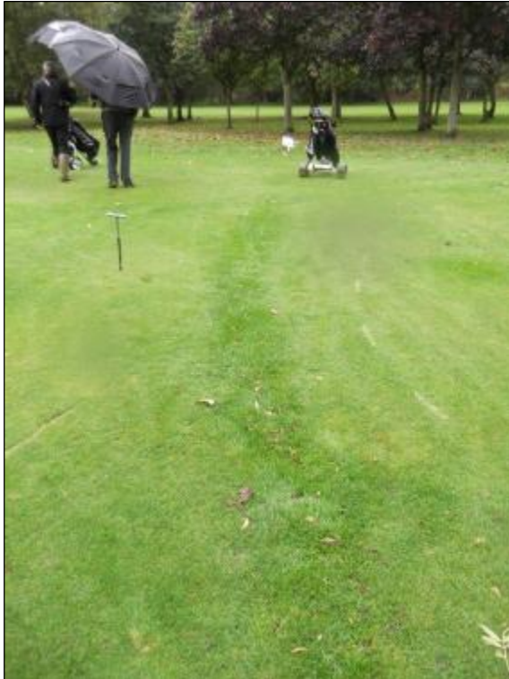
Photograph 5 – Sunken drain lines on 12 th approach in need of releveling.
